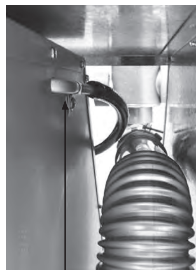
Flue condensate pipe connection
